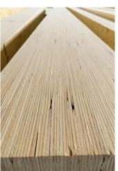
• Beams are glued both from full and jointed lamellae
